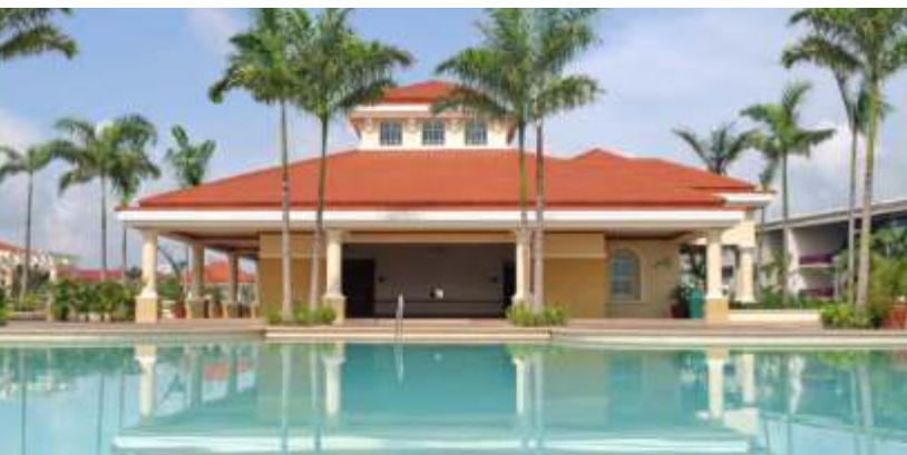
Brentville main clubhouse and pool
