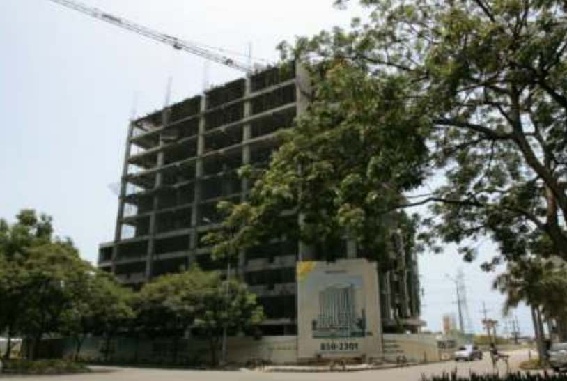
Construction of 2301 Civic Place in full swing
