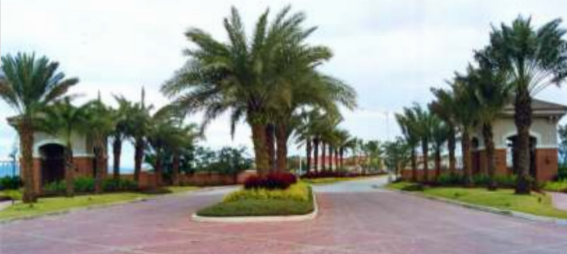
Brentville main entrance
